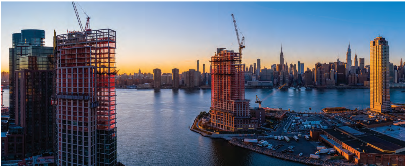
High-rise apartments under construction in Greenpoint, Brooklyn, 2021
